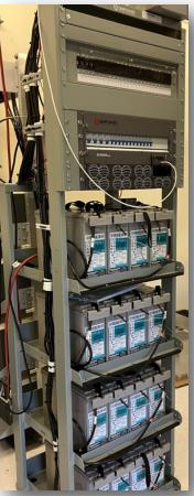
One Radio Network Operations Center (RNOC) provides the prime site control of the radio system and the interface to the State system. In the event that we lose contact with Columbus, the Radio NOC takes over and Warren County can operate in Site Trunking across our 9 tower sites, still maintaining local talkgroups. Each equipment rack is fed by two UPS power supplies, offering a high level of redundancy.
